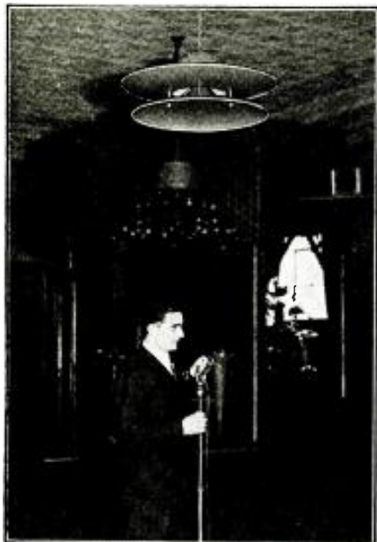
The "chandelier" speaker baffle installed in a typical dance hall directly over the spot from which the master of ceremonies makes his announcements.
